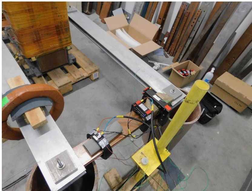
i) 3000/5A CT Photograph no. B26-20-AA-09E/04 Temperature-rise test
