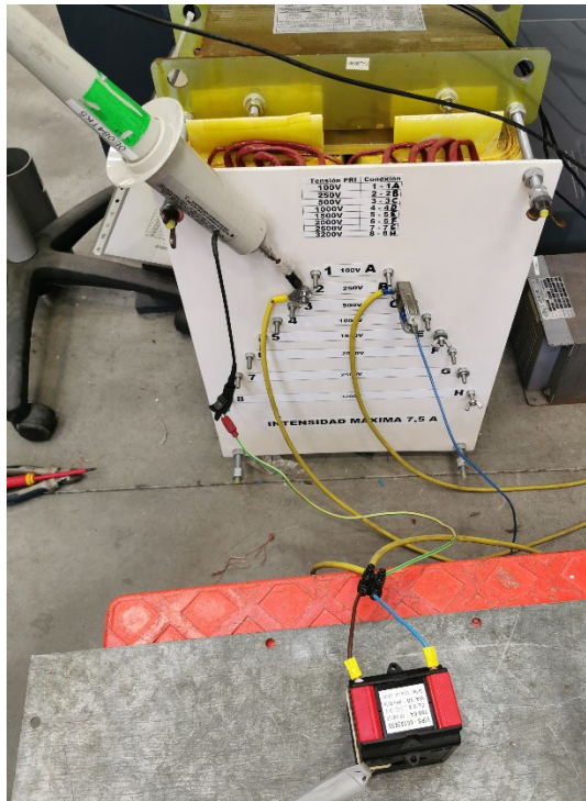
b) 200/5A CT Photograph no. B26-20-AA-02E/03 Inter-turn overvoltage test
