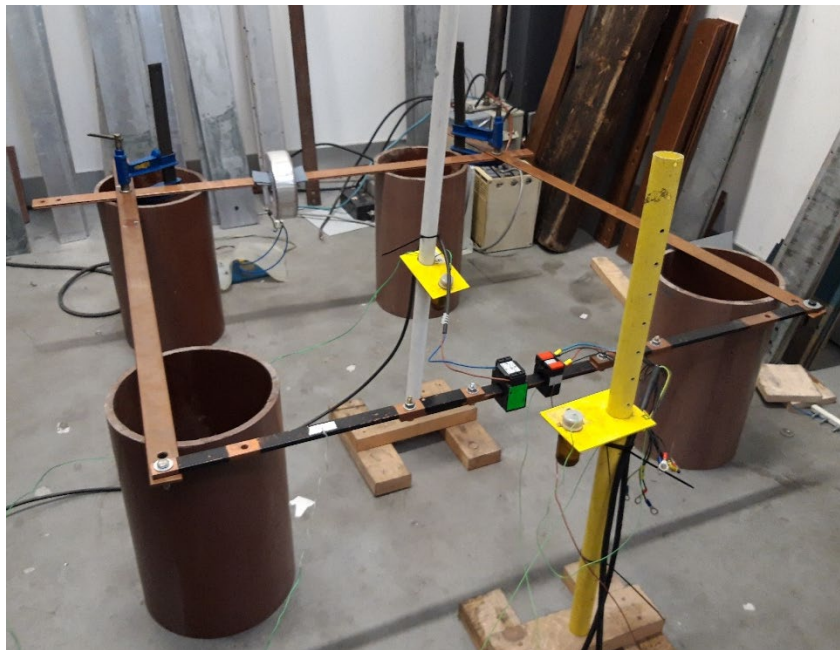
d) 400/5A CT Photograph no. B26-20-AA-04E/04 Temperature-rise test
