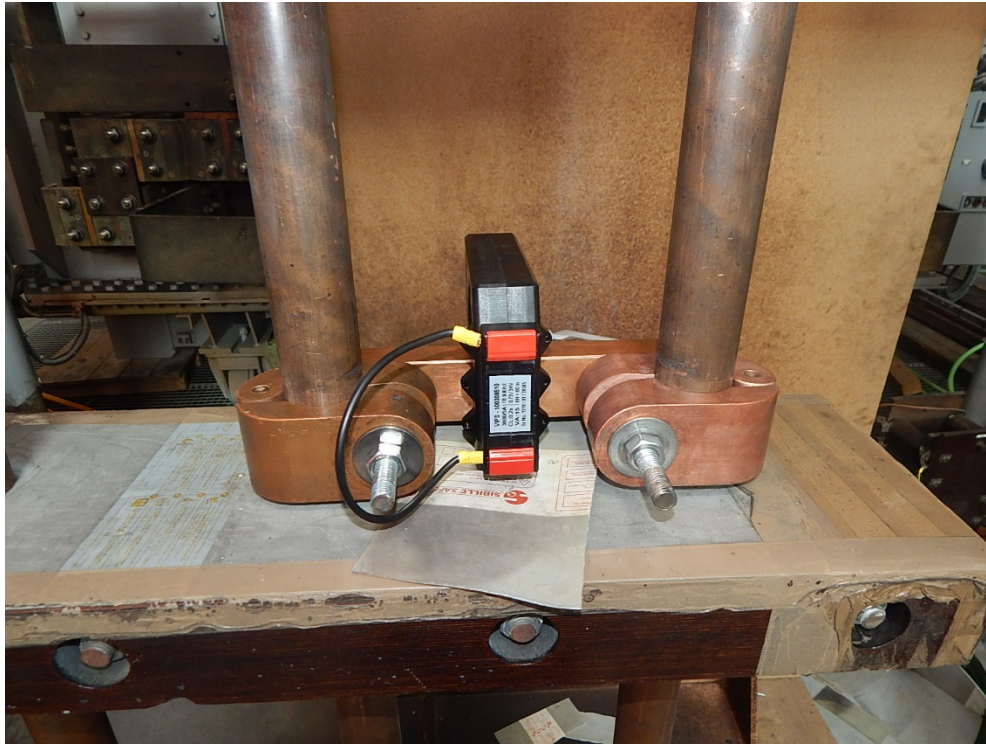
i) 3000/5A CT Photograph no. B26-20-AA-09E/05 Short-time current tests
