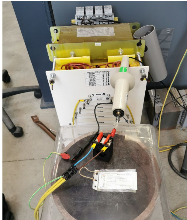
d) 400/5A CT Photograph no. B26-20-AA-04E/03 Inter-turn overvoltage test
