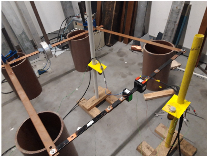
b) 200/5A CT Photograph no. B26-20-AA-02E/04 Temperature-rise test
