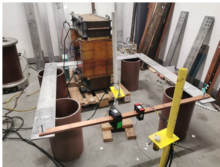
f) 1000/5A CT Photograph no. B26-20-AA-06E/04 Temperature-rise test
